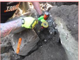
walls; the larger – the better in most cases. Large stones need to be solid and not move or wiggle after they are set. Thus BAR's offer more stability by their sheer weight and size. Chinking of small stones and dirt behind the step help even out the stone placement and provides firmness. Proper installation is required for a quality product that will be safe and long lasting.
