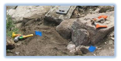
Before starting on any close-in rock work, all crew members in the immediate area will need to wear eye protection as a mandatory PPE (Personal Protective Equipment). Goggles or complete wrap eyewear is recommended due to the amount of rock shards that will fly in all directions.
